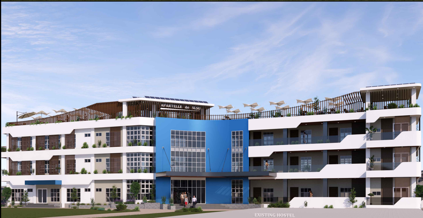
FRONT VIEW SHOWING HOSTEL BUILDING FOOTPRINT
